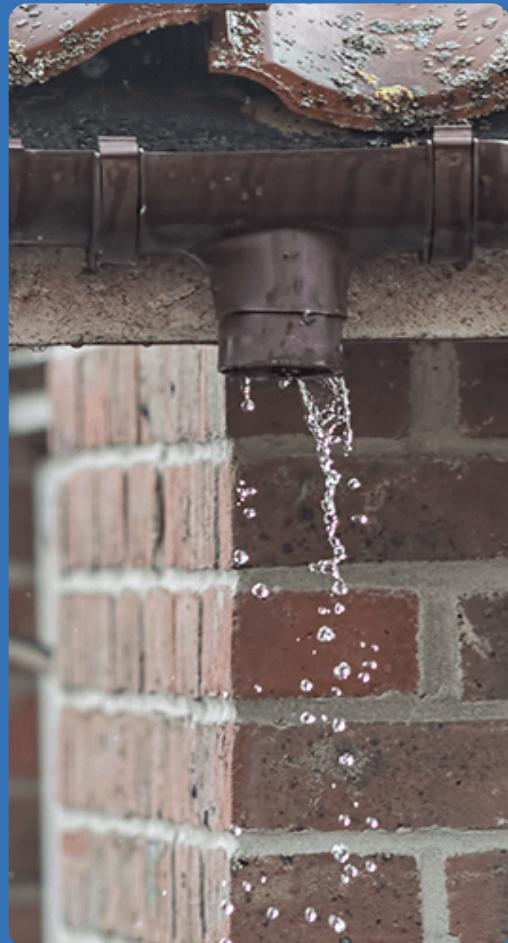
Penetrating damp is caused by water getting in from outside, often after heavy rain.
