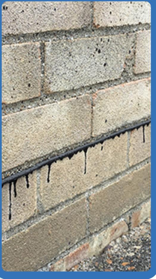
Rising damp happens when moisture from the ground travels up into the walls.
